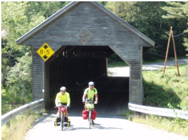
A covered bridge near Thetford, VT
